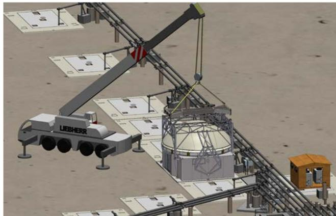
**Figure 15** - UT being installed at the Interferometer Array
