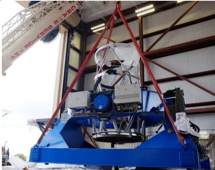
Figure 2 – Unit Telescope Mount being placed at the VCMF telescope pier
