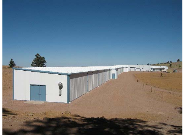
Figure 2: MRO Interferometry building at the observatory site.
