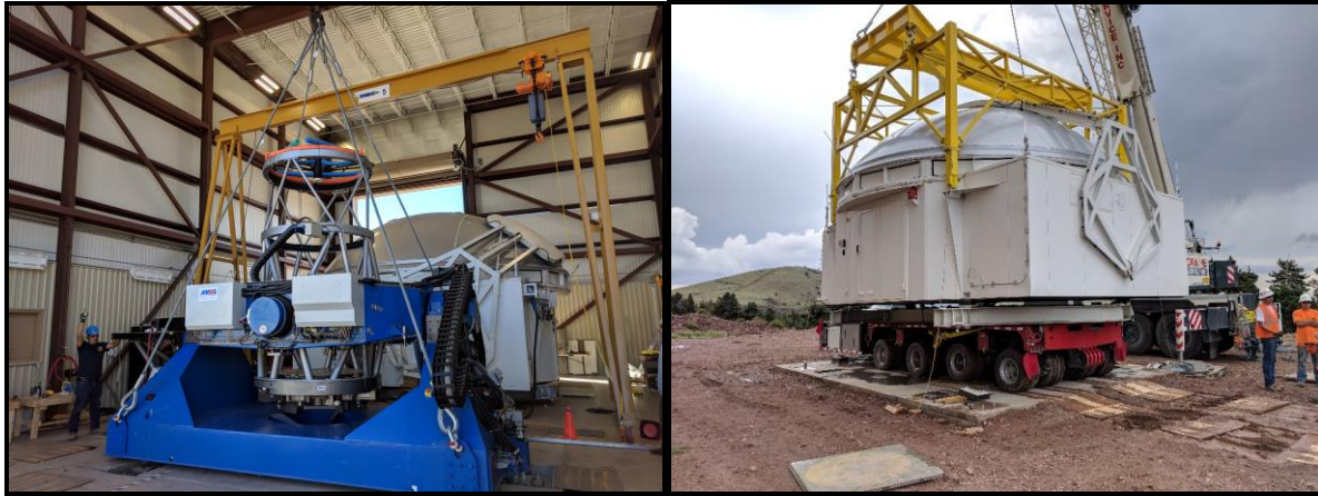
Figure 2a and 2b: At left is shown the lifting of the unit telescope mount (UTM) using a crane to place it on the integration station located outside the VCMF. In the background can be seen the unit telescope enclosure (UTE) ready to be moved as well. At right is shown the integrated UTM and UTE into one unit telescope (UT). The 28 ton UT was moved from the VCMF to the MROI array station on a leveling truck and placed on the kinematic pad using a crane with the custom lifting fixture instead of a reach stacker.
