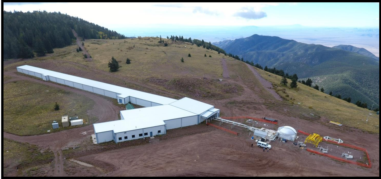
Figure 9: South facing drone photograph of completed beam combining and delay line facility for the MROI with the first unit telescope located on the west arm of the array. Next to the telescope is a temporary cooling system used to operate the telescope and electronics cabinets in UT#1. It is capable of supporting one telescope; the permanent system will have to be installed shortly. This will be located to the left, away from the array arms, in this picture. To the far right in the picture can be seen a yellow metal lifting frame used to assemble and relocate the telescopes.
