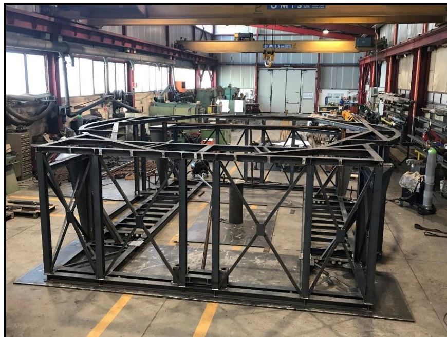
Figure 4: Metal skeletal frame of the lower half of UTE #2 seen in 2019 at the EIE Group facility in Italy.
