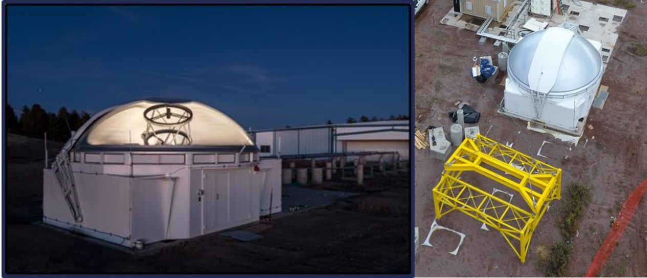
Figure 1: On the left is a night-time long-exposure of the first telescope in the MROI array positioned on the W7 foundation. The telescope, built by AMOS, can be seen inside the enclosure, built by EIE, via the internally illuminated structure. On the right is an overhead view of the same telescope seen next to the yellow lifting mechanism, which will be deployed during relocation of the telescopes between various foundations.
