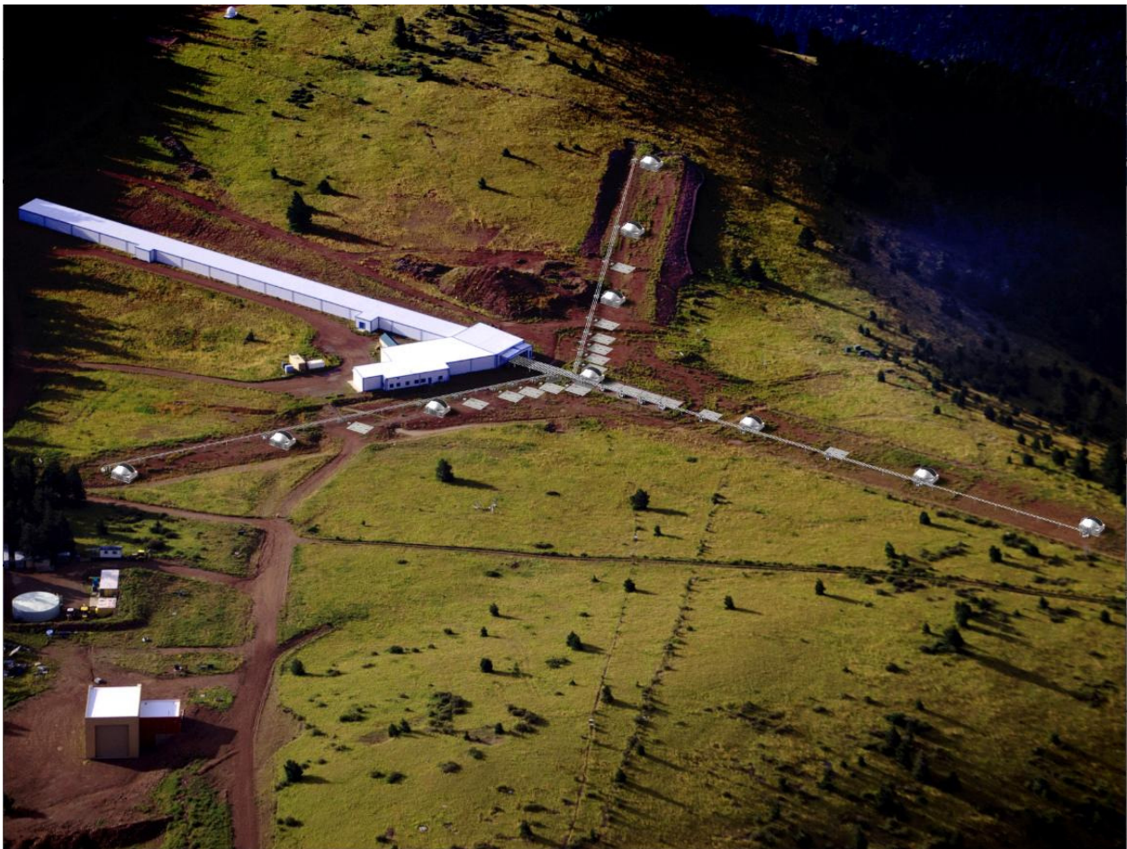
Figure 6: Artist's conception of completed MROI interferometer in extended configuration (everything except full array arms/pipes and telescopes are currently installed on site). The arm positions, labeled clockwise from the top of the picture, are S, W and N. Photo by Tyson Eakman.
