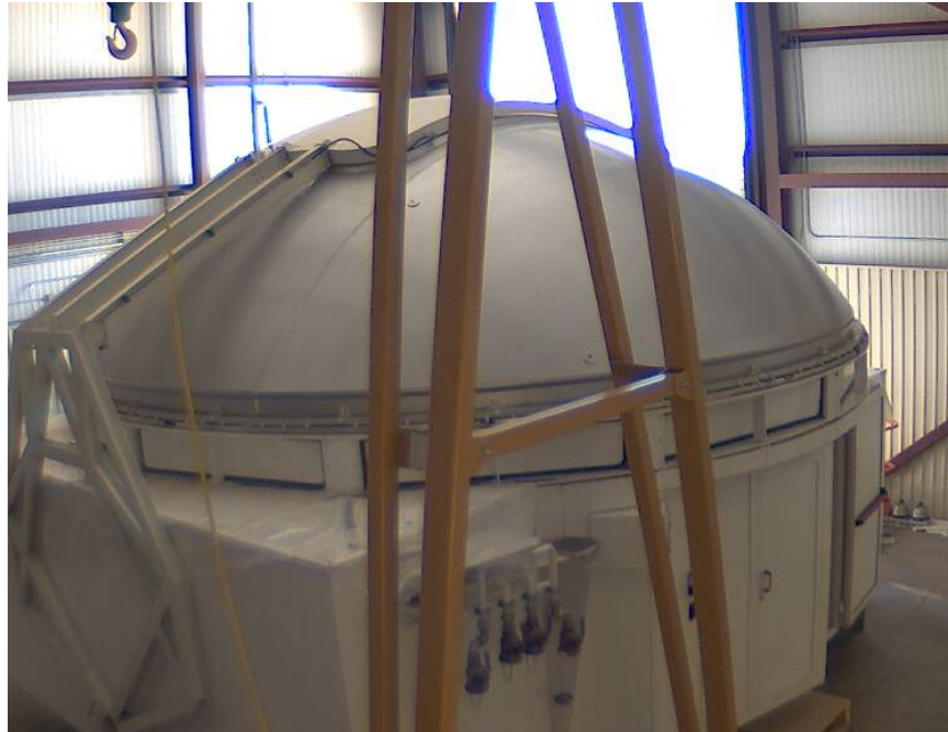
Figure 2: The first UTE under assembly in the maintenance facility at the Magdalena Ridge.
