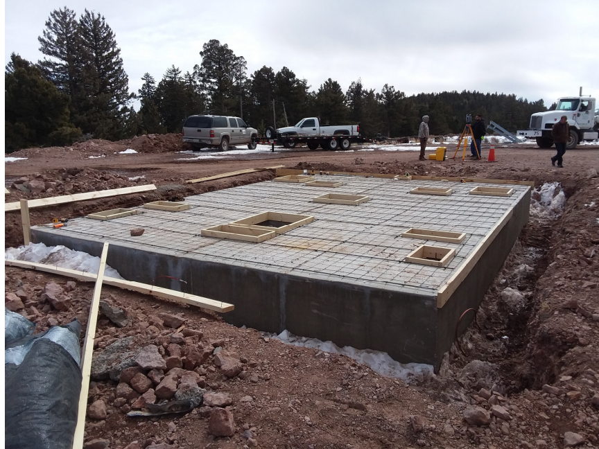
Figure 3: Integration station under construction located outside maintenance facility. The first UTM and UTE will be integrated on this station later this fall.
