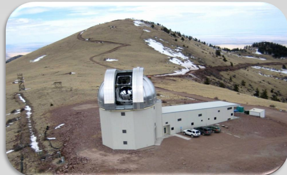
The MRO 2.4-meter Telescope (left): NESSI will be installed on the Nasmyth 'time mounting surface' port of the MRO 2.4-meter telescope sited in the Magdalena Mountains at an altitude of 3230m, about 48km west of Socorro – New Mexico. The telescope is a modified Ritchey-Chretien alt-azimuth design, capable of tracking targets up to rates of 10 degree/second along both elevation and azimuth axes.
