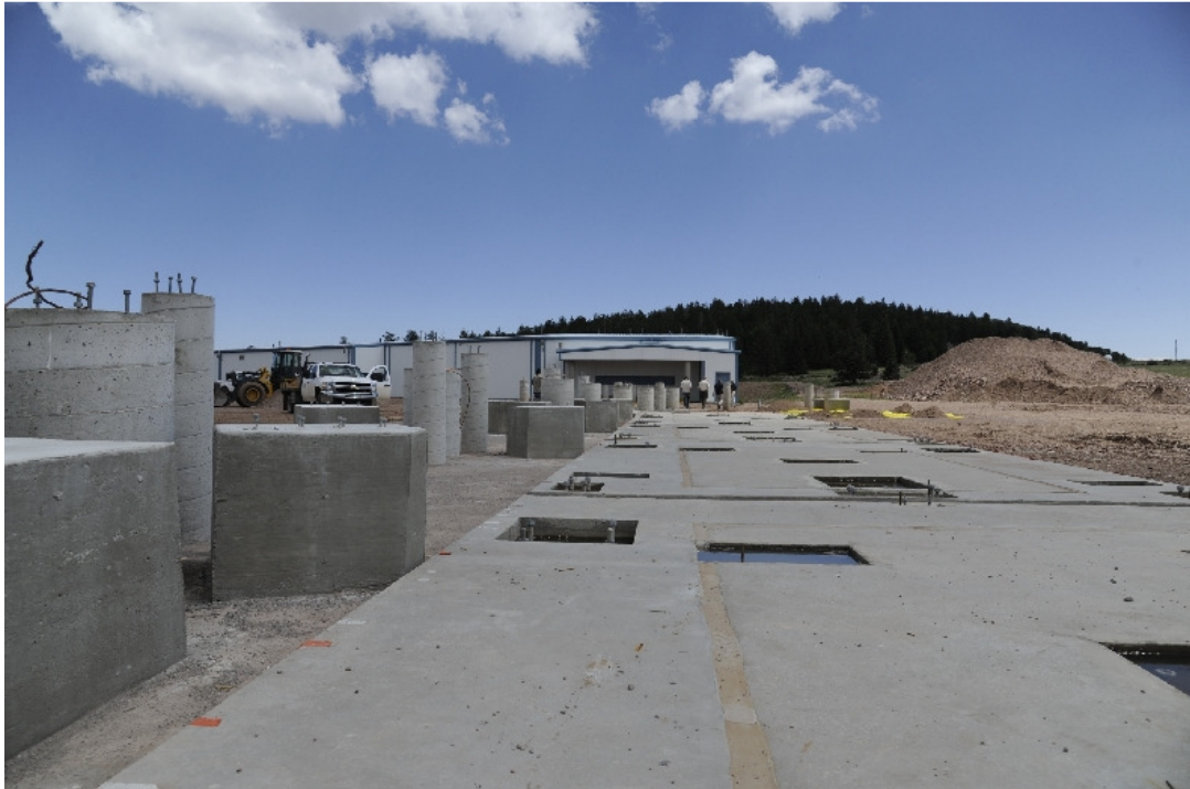
Figure 5: A view along the west array arm of the interferometer toward the beam combining facilities. Four of the telescope and enclosure foundations are shown together with the beam relay and vacuum can piers running along the left-hand side of the photo.
