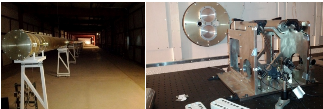
Figure 7: The current delay line pipe installation at MROI. On the left is the first 100m of delay line pipe for trolley #1 in the MROI beam combining facility, while at right is shown the metrology launch table within the inner beam combining area.
