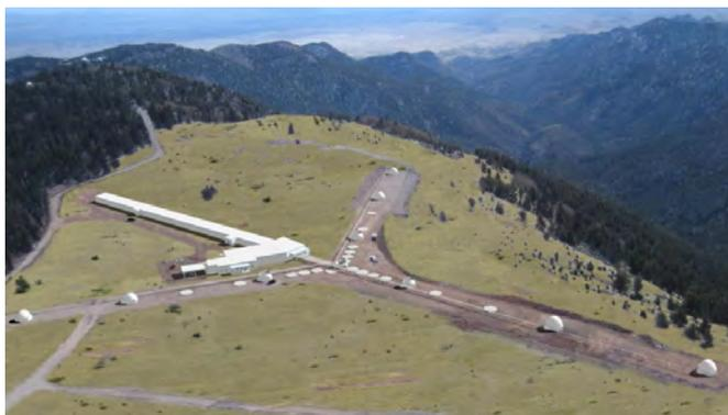
Fig 1: An artist's impression of the Magdalena Ridge Observatory Interferometer when fully deployed. In this figure the 10 telescopes are in their highest resolution configuration which gives a maximum baseline of  $\sim 340\text{m}$ . The long delay-line building to the left points roughly east.
