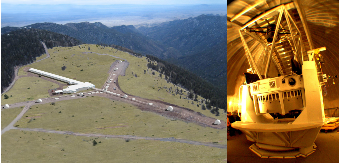
Figure 1. Two telescope facilities atop Magdalena Ridge. On the left is our architect's conception of the MROI facilities. The equilateral Y configuration with 28 pads is clearly visible to the right of the interferometric buildings. On the right is the fast-tracking 2.4m telescope which is now in operations.
