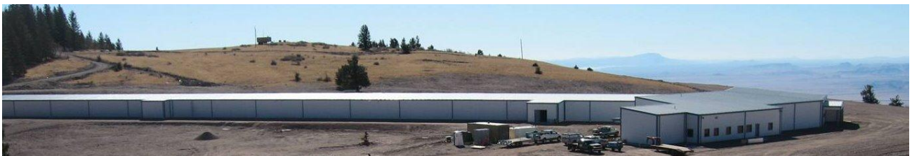
Figure 2. The beam combining and delay line facilities for MROI. Note the 200m long portion of the building extending off to the left, which houses the delay lines. Beams enter the building from the center of the array arms on the right side of the photograph.
