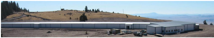
Fig. 6 A recent photograph of the MROI beam combining facility. To the left in the photograph extends the single pass delay lines in a 190 m long building. To the right in the photograph is the location of the center of the array arms to be laid out in an equilateral-Y with the longest baseline attaining nearly 345 m (adapted from Creech-Eakman et al. 2008)
